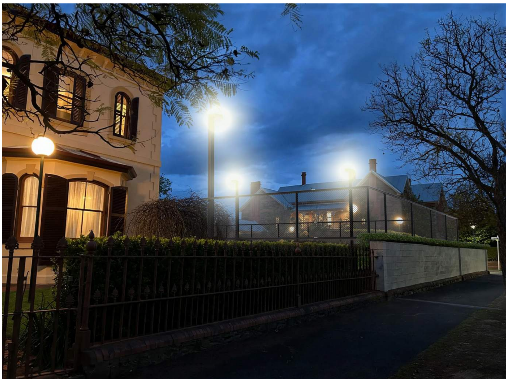
After: west approach, night.
