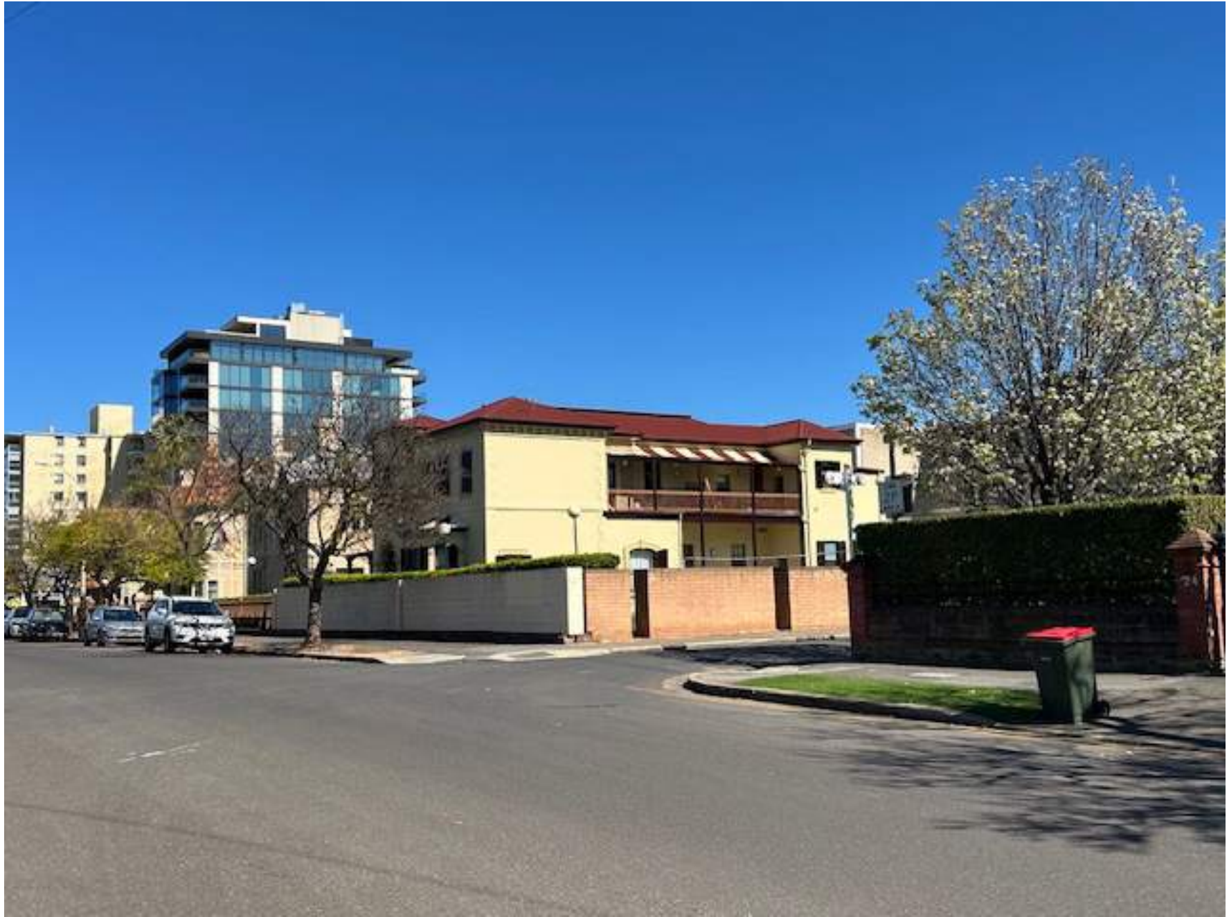
Before: corner view, day.
